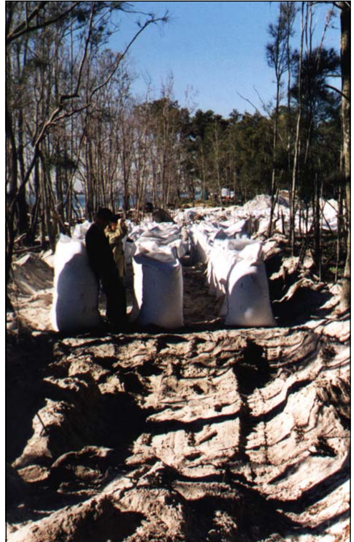
ELCOROCK® containers filled, waiting for placement
