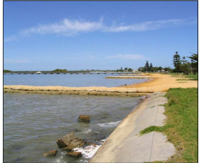
Old protection vs new protection
