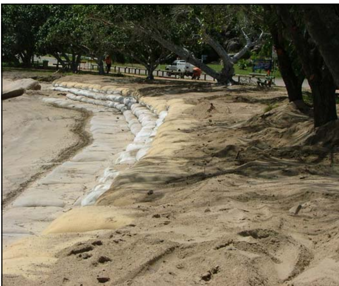
After construction of the wall and backfilling
