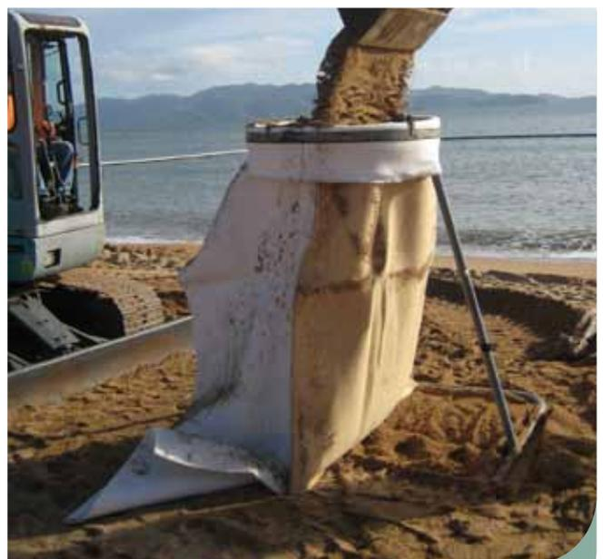
Figure 2. Filling sand container
